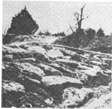
Veterans Lake Spillway Repairing first erosion drop
