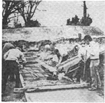
Veterans Lake Spillway 3-9-84 Repairing first erosion drop
