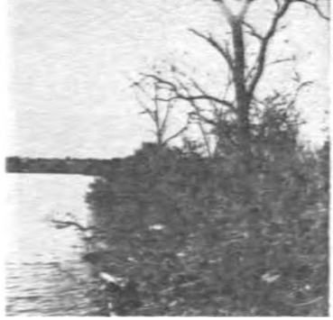
Veterans Lake Dam Clearing brush & trees
