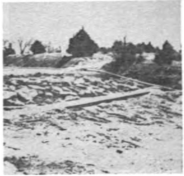
Veterans Lake Spillway Repairing first erosion drop
