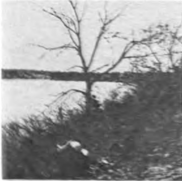
Veterans Lake Dam Clearing brush & trees
