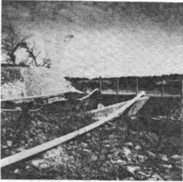
Veterans Lake Spillway Siphons + Pump
