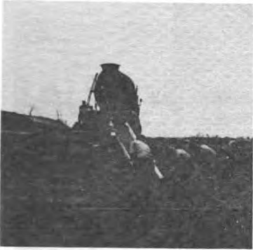
Veterans Lake Spillway 3-9-84 Repairing first erosion drop
