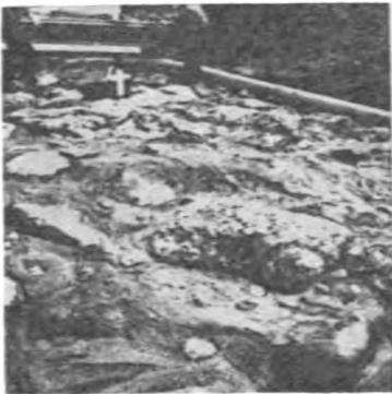
CHICKASAW NRA 2/29/84 ROUTING ROCKS SET IN spillway
