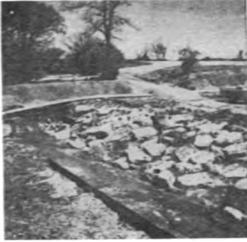
Veterans Lake Spillway Repairing first erosion drop
